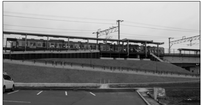
The ramp for access to the elevated platforms.
