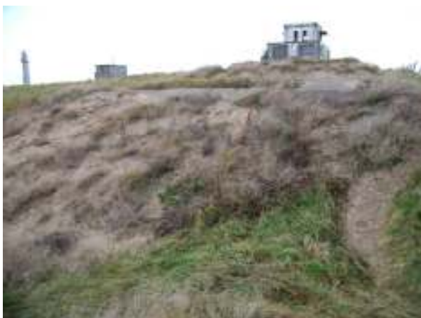
The crew bunker for 15 men, Regelbau 656, in January 2007. (F Philippart)
