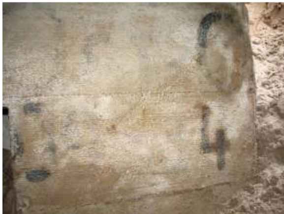
The bunker has been stripped of all its equipment but...
