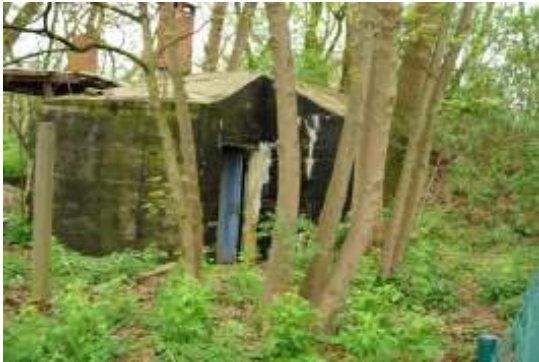
The bunker at the Westhoek domain.
