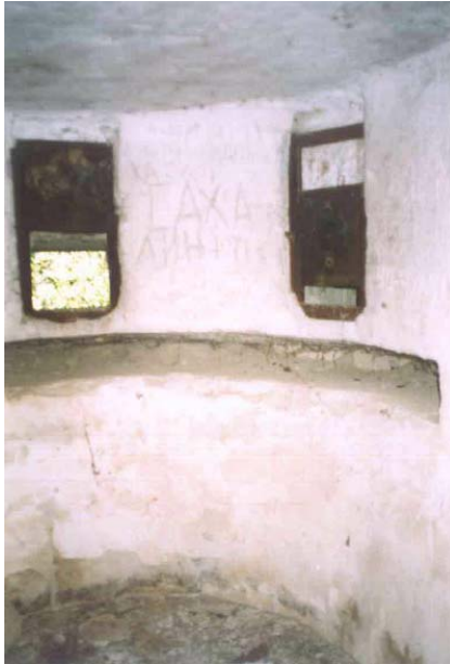
Inside view from 2 fire positions
