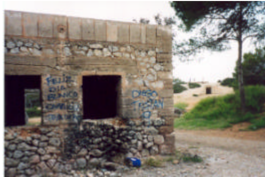
Barracks and tunnel entrance.
