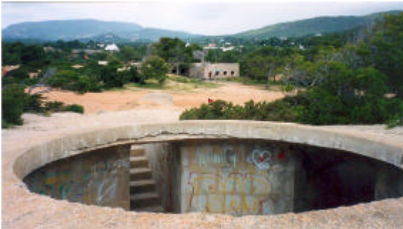
Gun 1 and roof of the tunnel
