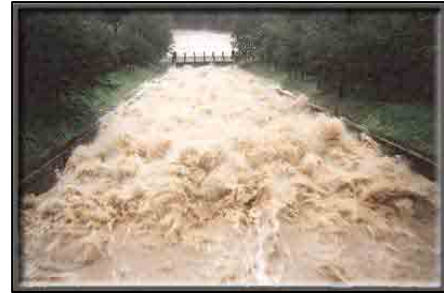
Illustration 02: A dam channeling out flood water [6]
