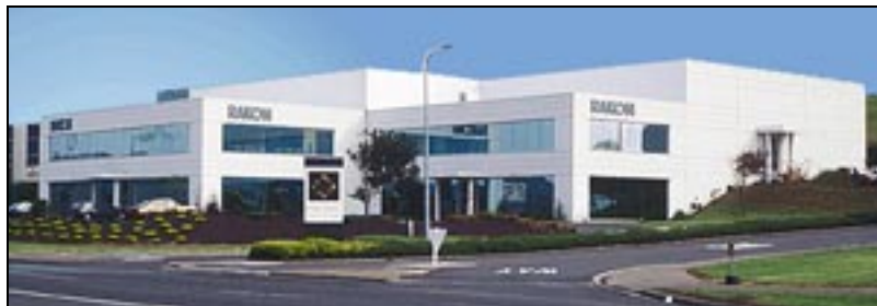
Figure 01: Rakon's Auckland Production Facility
