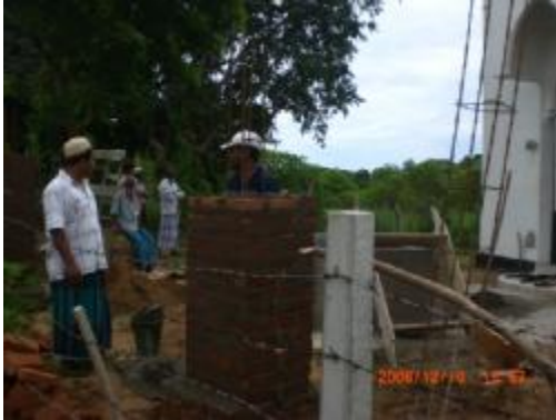
Construction being supervised by Mr Roy Marso – Committee member And project coordinator.
