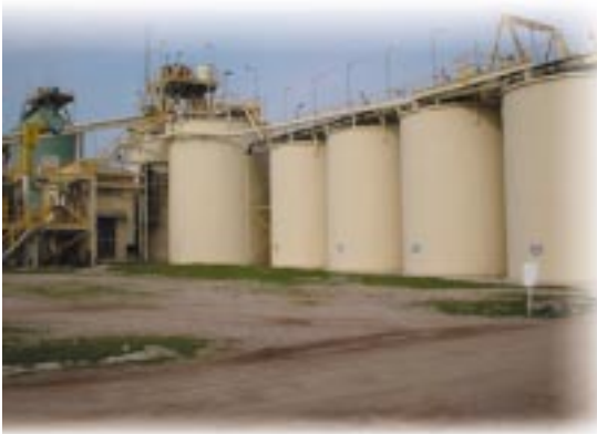
LEACH ABSORPTION TANKS AT OVACK MINE.
