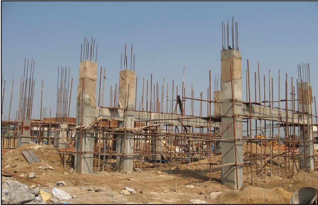
RCC STRUCTURE FOR BOILER 1
