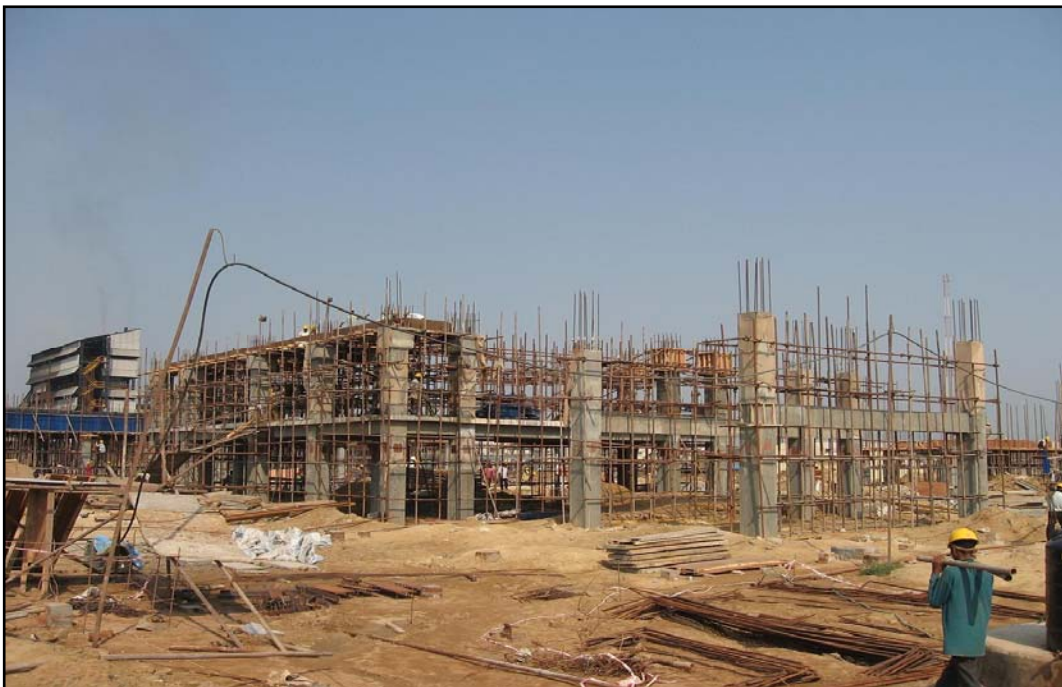
RCC STRUCTURE FOR BOILER 2
