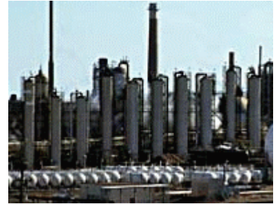
Photo courtesy Phillips Petroleum Distillation columns in an oil refinery
