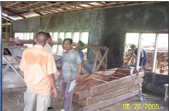
On-going replacement/repair of four (4) classrooms in Lower Tungawan Elementary School. Mr. Expedito Bejerano of DepEd joined the team in the inspection.
