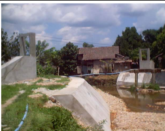
Superstructure of the uncompleted Handina Bridge
