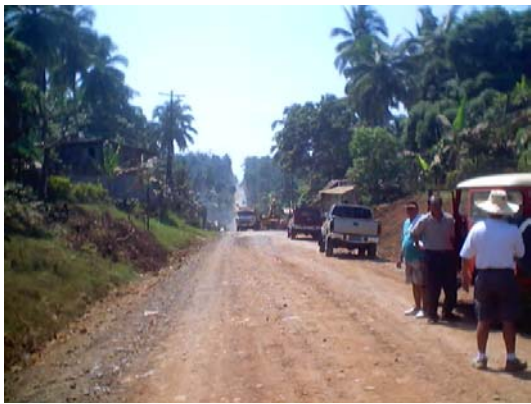
On-going rehabilitation of Aurora – Monte Alegre Road
