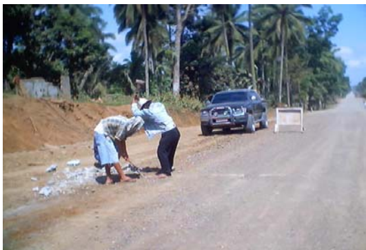
Relocation of water pipe
