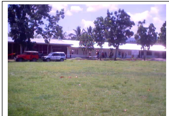
Rehabilitation of Seven (7) Classroom
