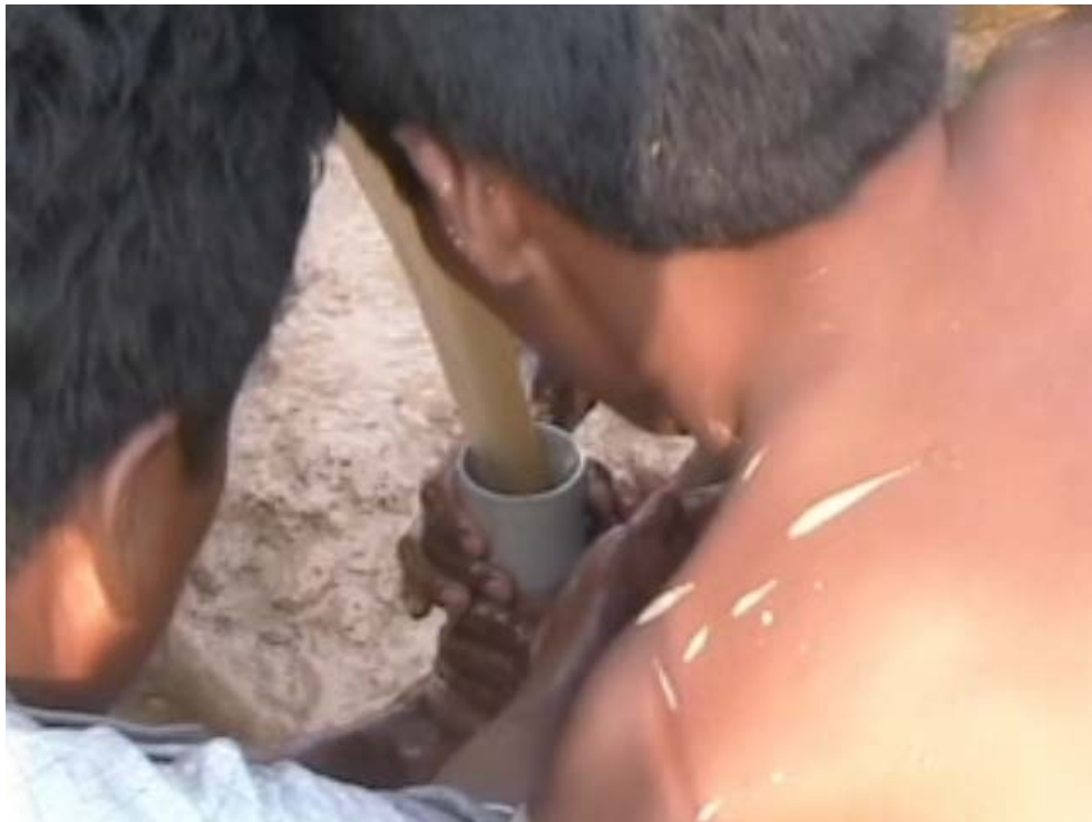
Adding water to each section of casing to counter weight the buoyancy of the mud in the hole. Water is added to each section.
