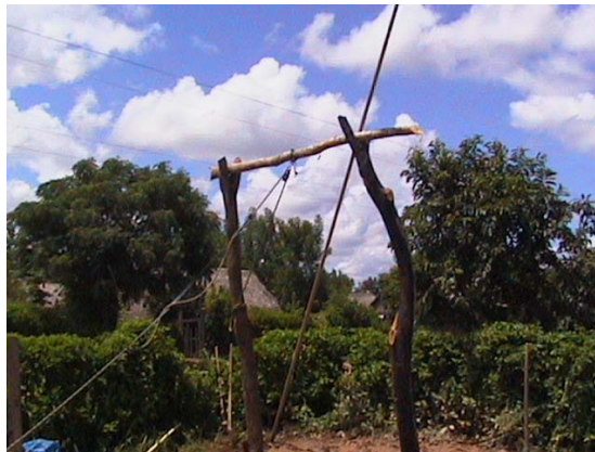
The “derrick” set up with 6 meter long drill tool leaning against it.
