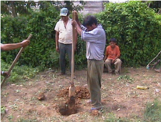
Digging the Pilot hole.
