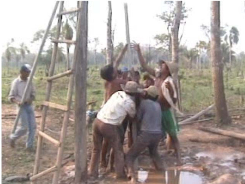
Casing the well
