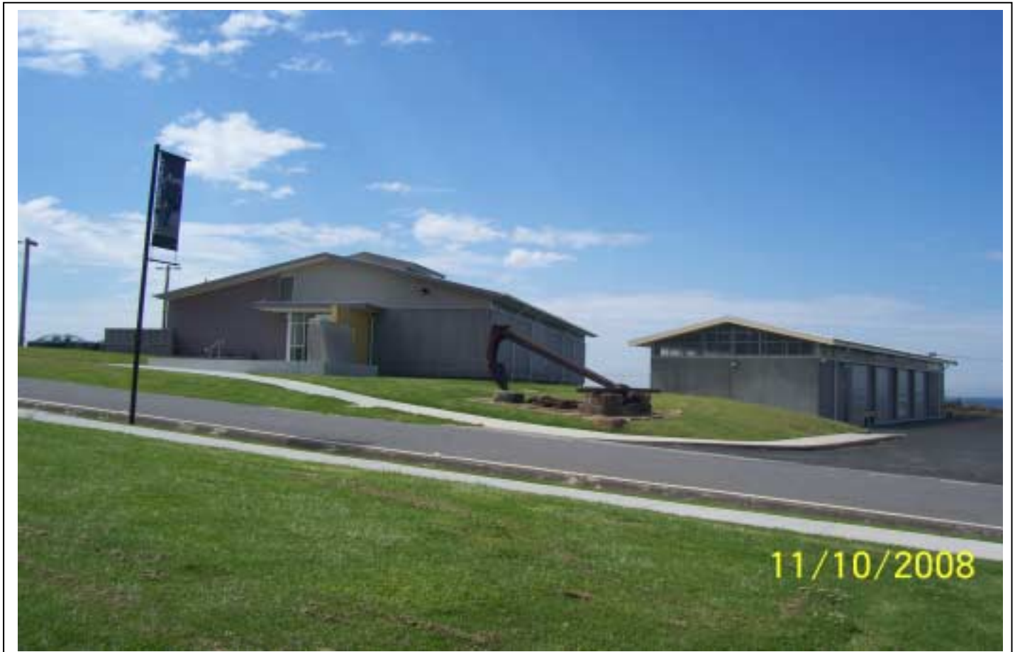
Below: Two buildings recently built without a Newcastle City Council Development Application or Development Consent
