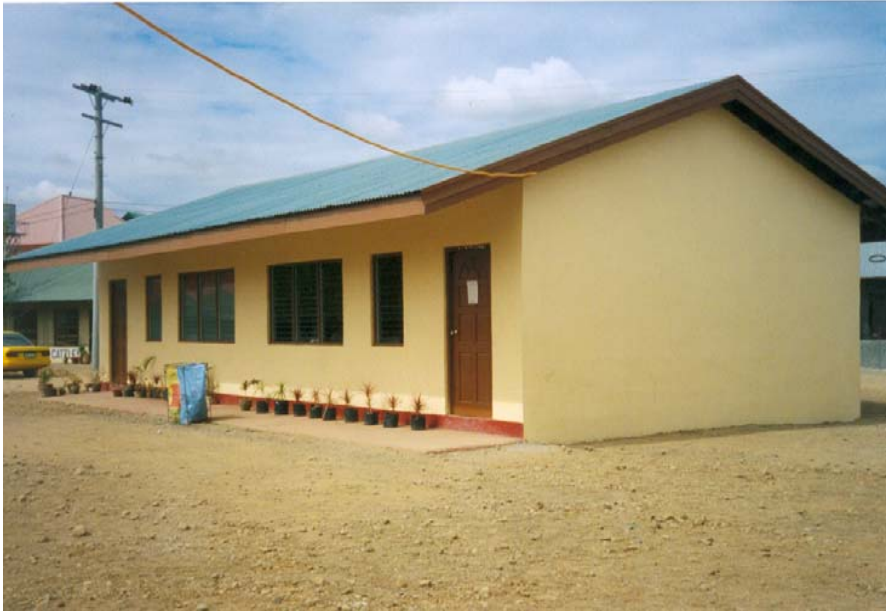
COMPLETED 2-CLASSROOM BUILDING NEAR THE REAR GATE OF PHS WHICH WAS SOLICITED BY FEPJAAF FROM THE FILIPINO CHINESE CHAMBER OF COMMERCE –CITY OF SAN FERNANDO(P) CHAPTER.
