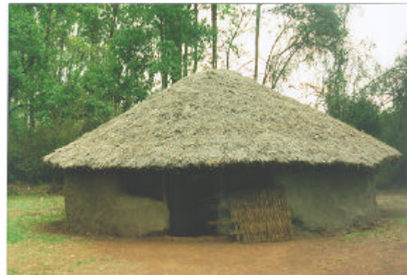
Fig 3 Luo Traditional House (Note the mud walls and the grass-thatched roof)
