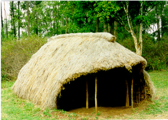
Fig 4 Taita Resting Hut Note the thatch throughout the building
