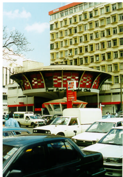
Fig6 Chai House, Nairobi
