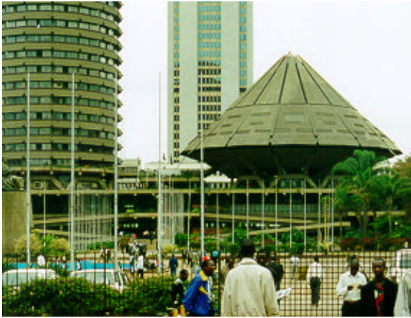
Fig 7 KENYATTA INTERNATIONAL CONFERENCE CENTRE Note the "hut" on the podium
