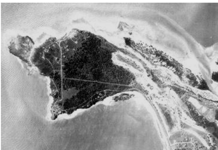
From the air: East Point in 1955. Note that Lake Alexander did not yet exist; note also the golf course fairways extending from the current site of the Lake north-west into areas that are now regenerating vine-thicket.
