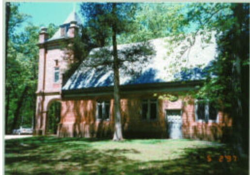
St. Peter's Parish Church, front and side views
