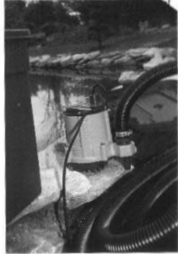
Thread the lid onto the base that is affixed to the pump inside the container. Photo by H. Nash.
