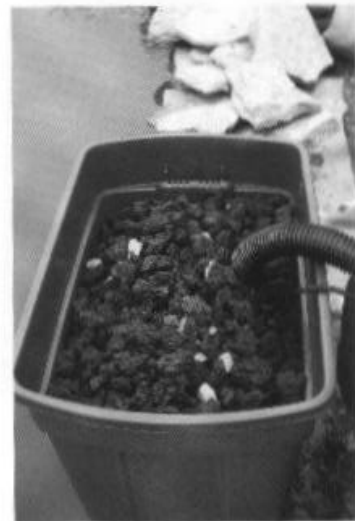
Fill around and over the pump with washed lava rock. Photo by H. Nash.
