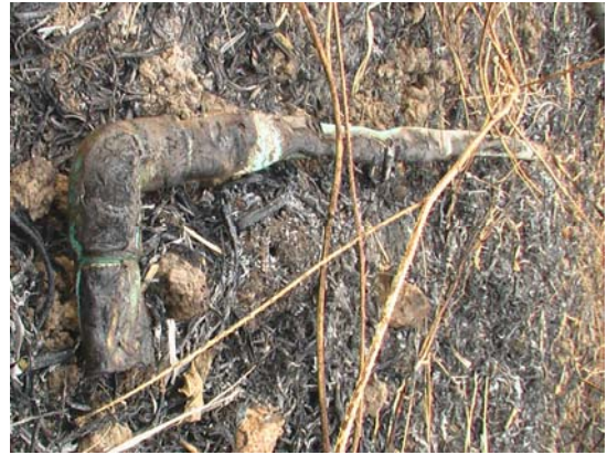
The unused water pipe from the dam to cultivation
