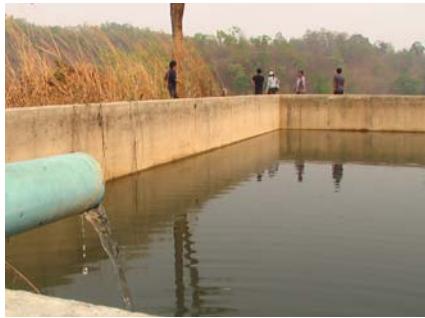
Water from this dam is supposed to use for cultivation at Huai Ja Kan but unfortunately the dam is lower than the level of cultivation area.
