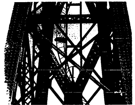
5b. Viaduct at Garabit (1880-84), Gustave Eiffel, detail.
