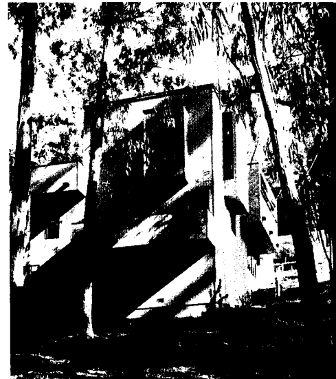
The Graham house in Berkeley, California, by Richard Peters and Peter Dodge (above) The Cary house in Mill Valley, California, by Joseph Esherick (opposite)
