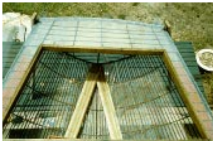
2 layers of 5mm sq. mesh outside and 1 inside.
