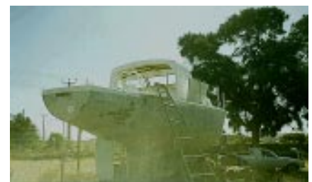
Unveiled! The join is very fair and will be invisible when painted.
