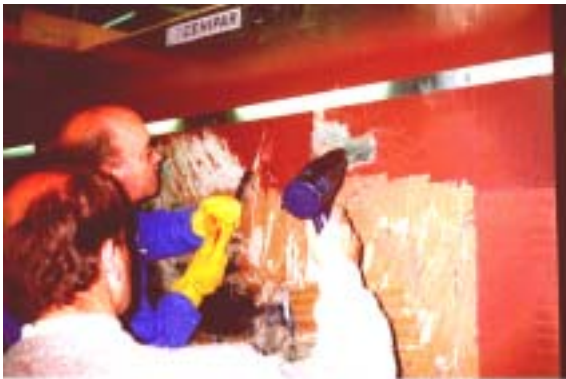
Figure 3.24. The removal of the Tin-free SPC by blowing hot air and gently scraping the surface.
