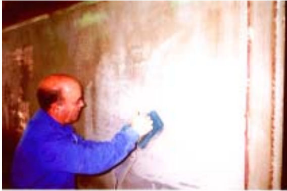
Figure 3.26. Sanding of the surface.
