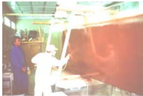
Figure 3.22. Application of the first coat of Tin-free SPC.
