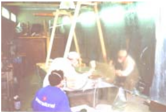
Figure 3.21. Application of the primer.
