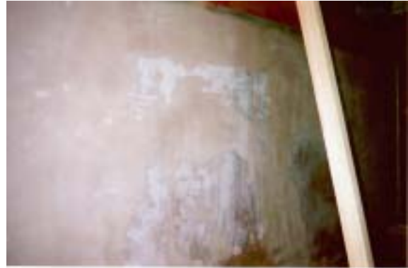
Figure 3.27. The surface after sanding.
