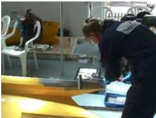
Figure 3.45. Application of the Foul Release tiecoat.
