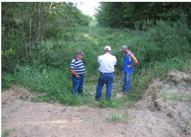
GPICES board members pictured below are meeting with a contractor to discuss completion of a low water crossing.
