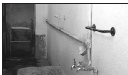
Hand rails nailed on the wall
