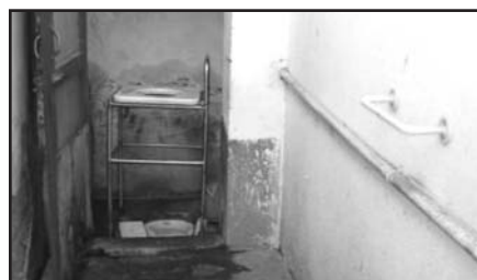
Toilet after modification
