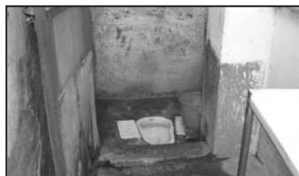
Toilet before modification
