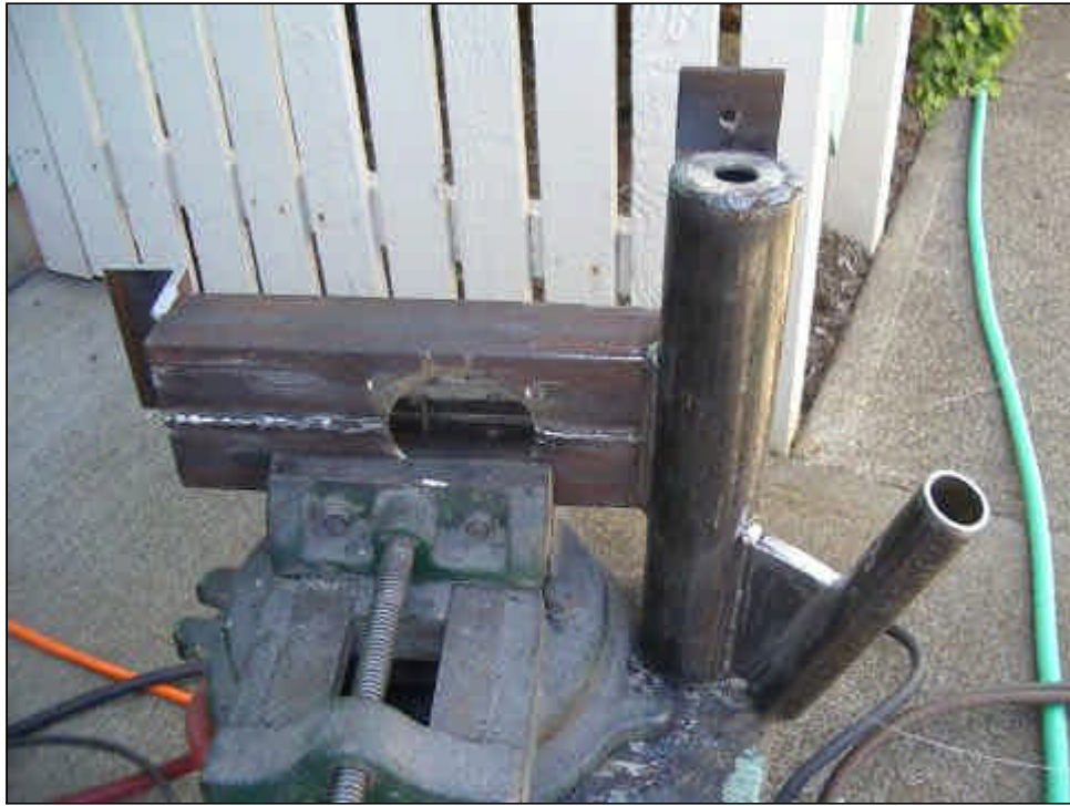
Hub carriage. The pipe on the left is the tail vane hinge.
