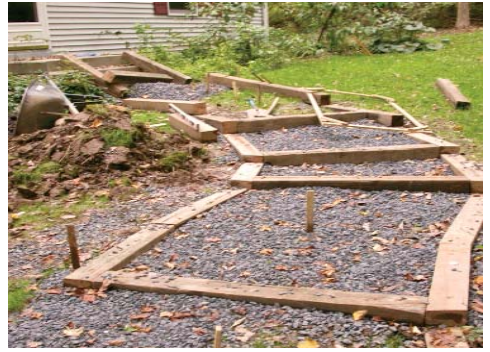
Terraced path to front door under construction.
