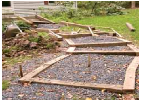
Terraced path to front door under construction.
