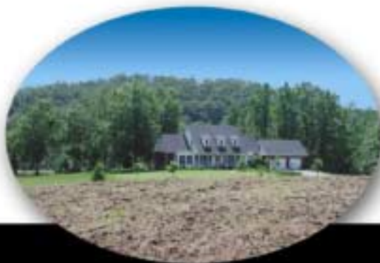
Fig. 5. On the wooded ridge behind the farmhouse, the Fort Payne Chert aquifer lies just beneath the soil, making this an ideal recharge area for clean water.
