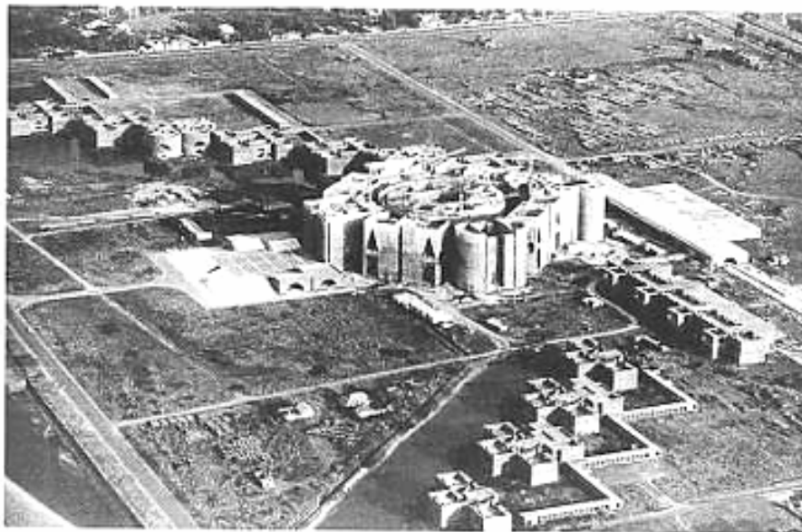
Figure 6: National Assembly Complex during construction. (source: Gast, 1999)
