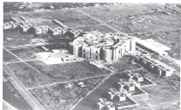
Figure 01: Capitol Complex during construction.
