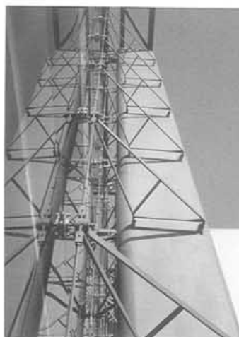
2.12 Financial Times building, London (architect: Nicholas Grimshaw & Partners)
