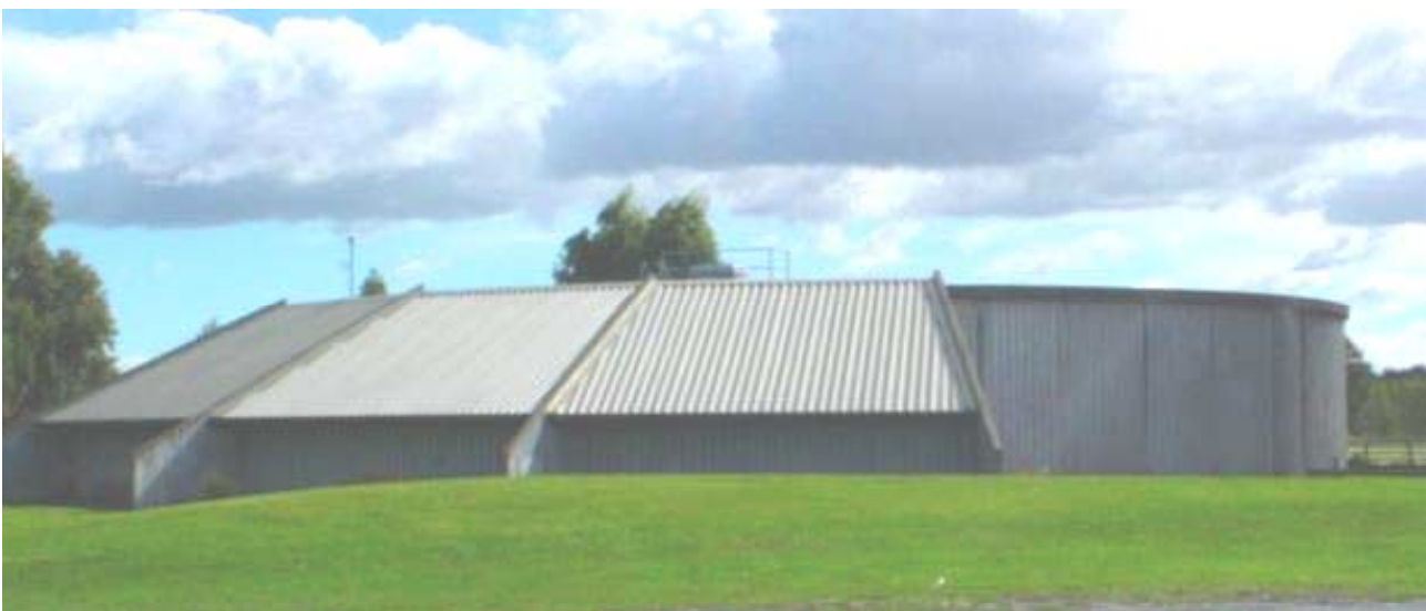
Reservoir and pump station constructed at Halswell in 1990
