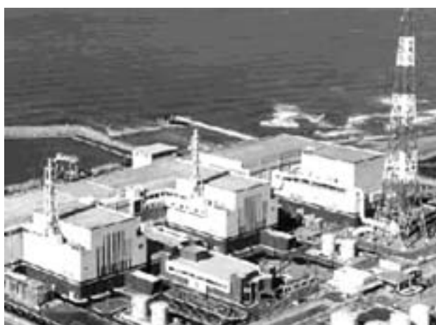
Figura 5. Central nuclear de Kashiwazaki-Kariwa
