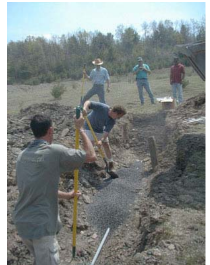
spreading limestone
