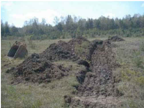
ditch for lysimeter
