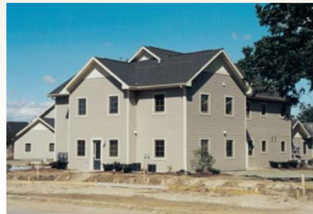
Construction of the Genesis East Apartments in southeast Grand Rapids will soon be completed.
