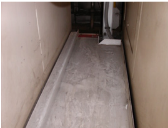
FIGURE 6. OPEN SLOT INSIDE THE CAR IDENTIFIED FOR HOUSING DATA RECORDER AND UPS UNIT
