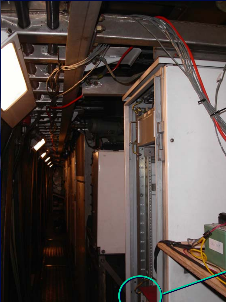
Wire Runs Between Transducers and Recorder Inside the Power Car
