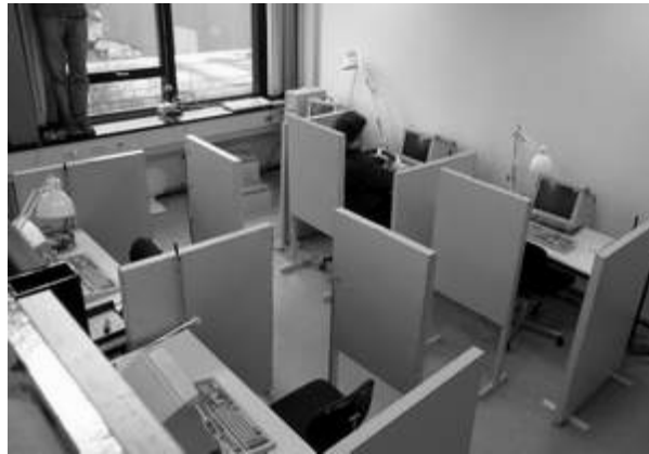
Figure 2.9 Overview of the field lab with workstations and radiant panels installed.
