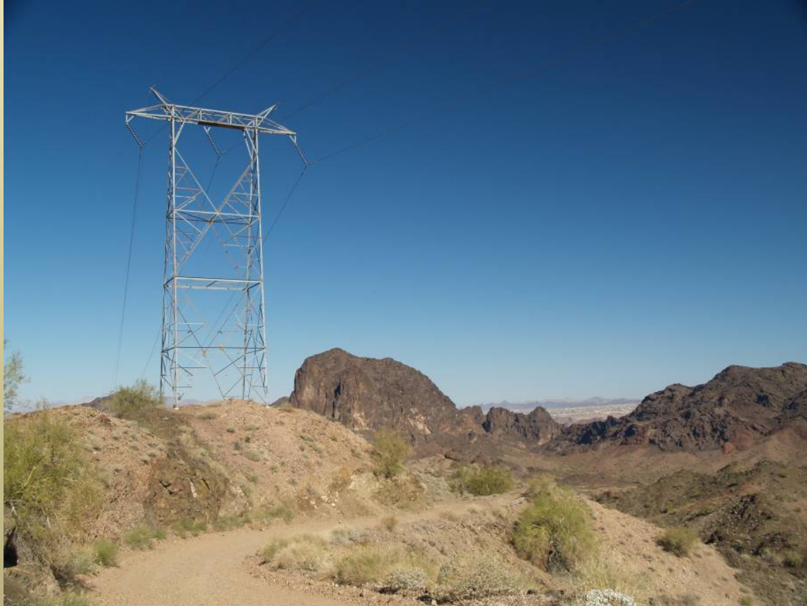
An existing angle tower northwest of Parker
