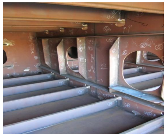
Figure 3: Ballast section steel preparation
