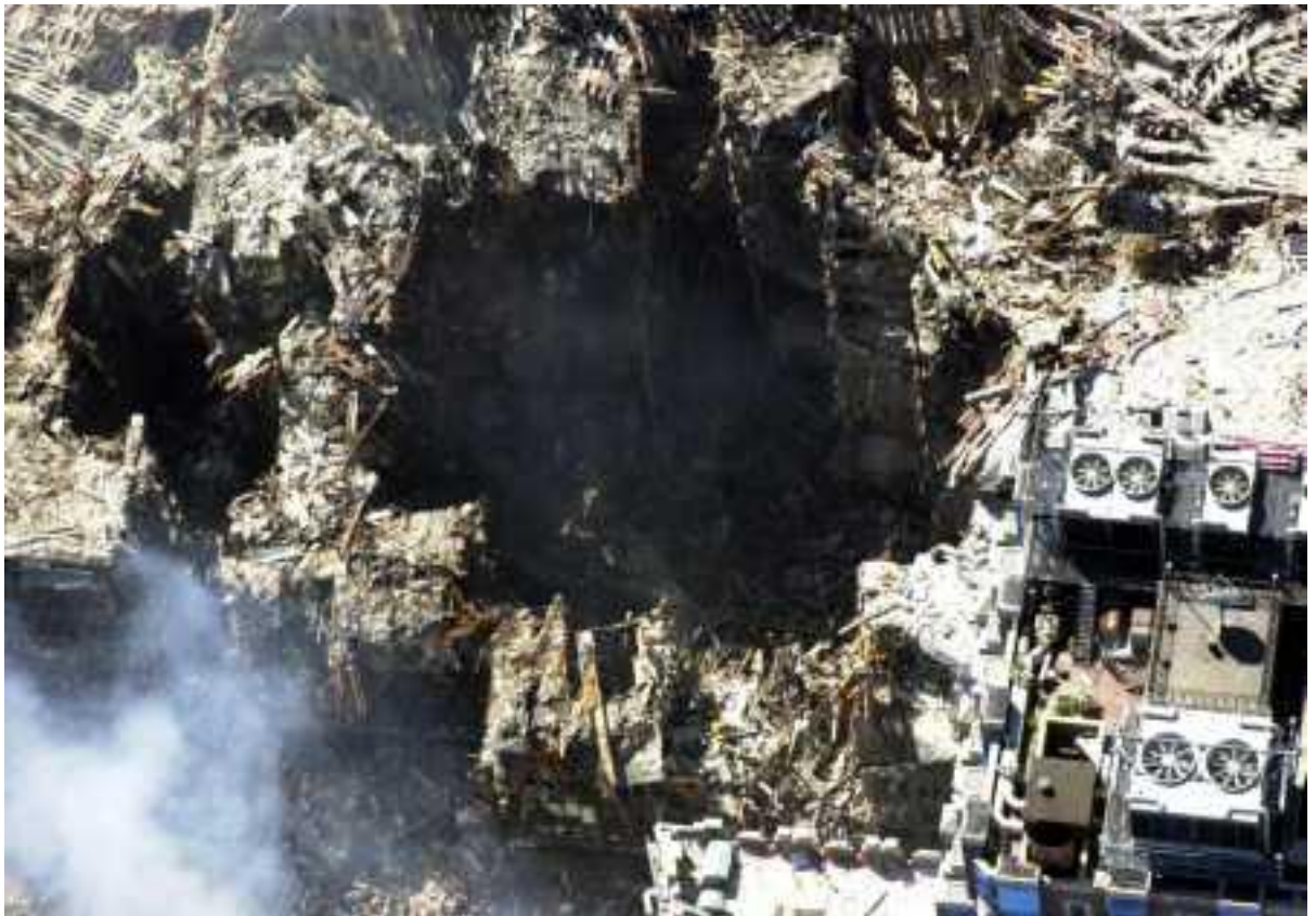
Fig. #L3: The above photograph for me personally is a symbol of how uninformed (if not intentionally misled) are people of the Earth. This photograph shows an underground "tunnel" that after the "collapse" of WTC buildings in New York, appeared in the place where previously stood one of these buildings - i.e. the one which was NOT hit by any airplane. But in what strange manner this building needed to "collapse", that instead of a pile of rubbles sticking high up, it left a tunnel in the ground? Or, perhaps, it was not a "collapse" at all, but an evaporation of this building carried out in such a manner that it "simulated" the evaporation by a UFO vehicle
