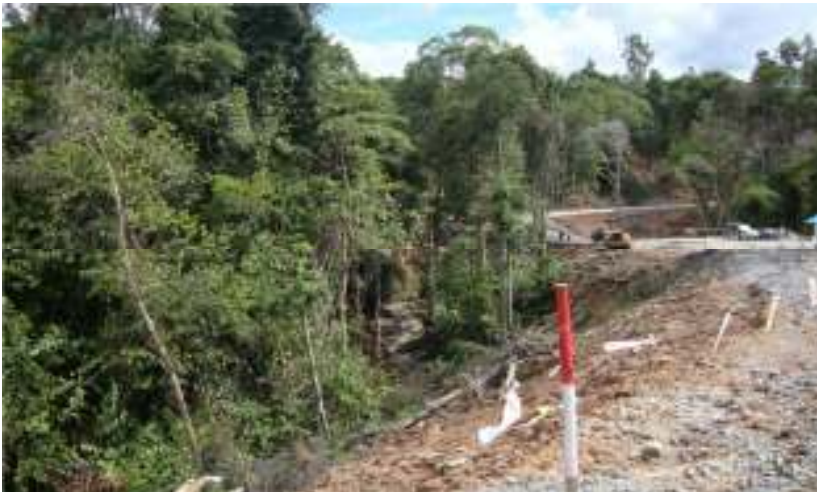
Date : 25-Sep-10 Description : Zone C P2 Overall view.
