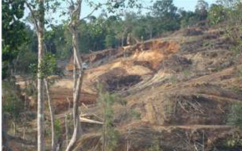
Date : 25-Sep-10 Description : Zone A P9 Site clearing at Sub-zone A2.
