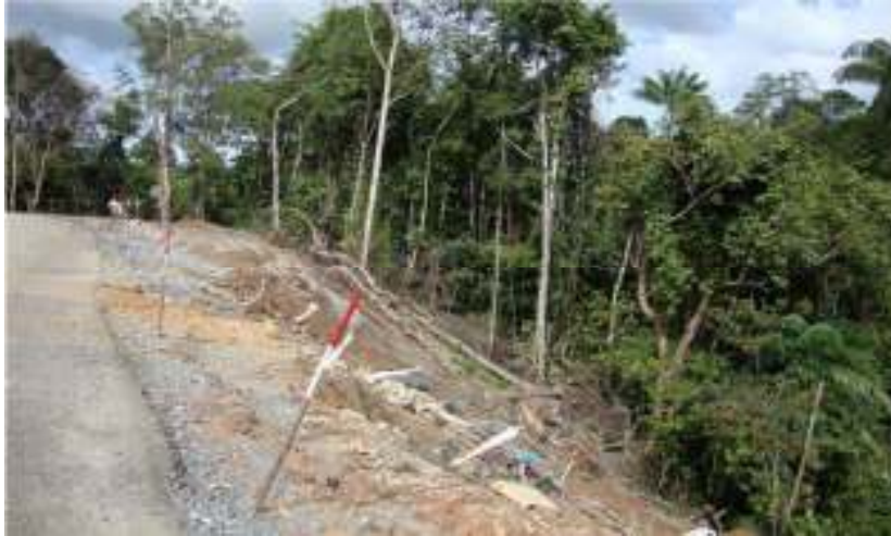
Date : 25-Sep-10 Description : Zone C P1 Overall view.
