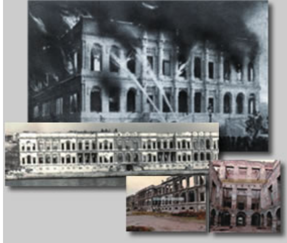
The Ciragan Palace in Istanbul after it was burned and its interior design and decorations destroyed. Someone looking at the palace in this condition could never fully imagine how magnificent it had once been.
