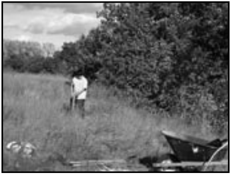
Researcher Dr. Kawano builds a concrete structure for the Japanese developed magnetometer.
