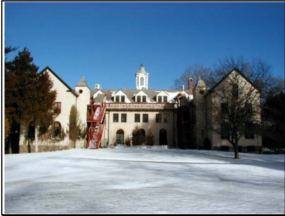
Building 1 – Founders Hall
