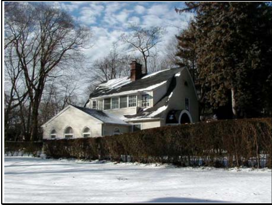
Building 15 – Washington House
