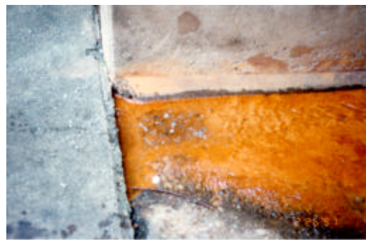
b) Piping on spillway flood
